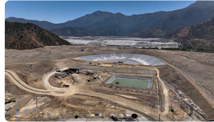
Hydraulic dewatered stacking (HDS) is an emerging technology that allows the safe disposal of mining by-products and accelerates our progress towards the end of wet tailings storage. Featured is the demonstration plant at our El Soldado copper operation in Chile, where HDS technology is being trialled on a large scale.
