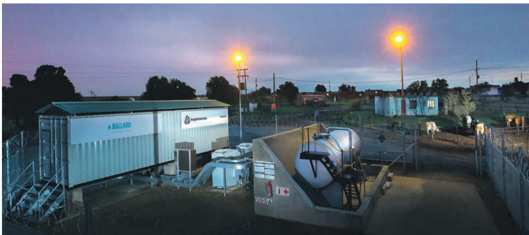
Anglo American Platinum's fuel cell installation at Naledi Trust supplied power to 34 homes in the village, pictured in the background
