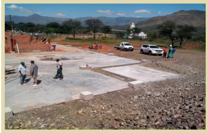
Construction of new facility
